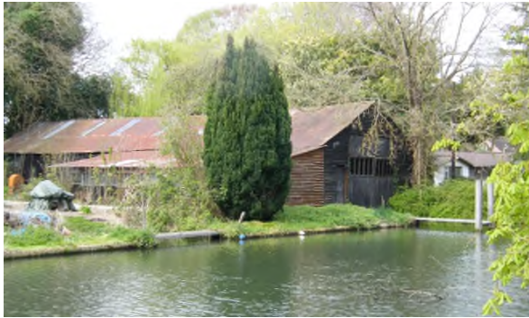
The historical boatyard and workshop building
