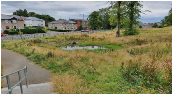
Flood detention pond in Croft Park Avenue
